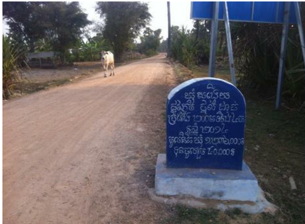
- Road construction (made from white soil) implemented 2014
