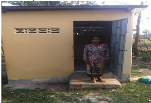
- 161 families had toilets
