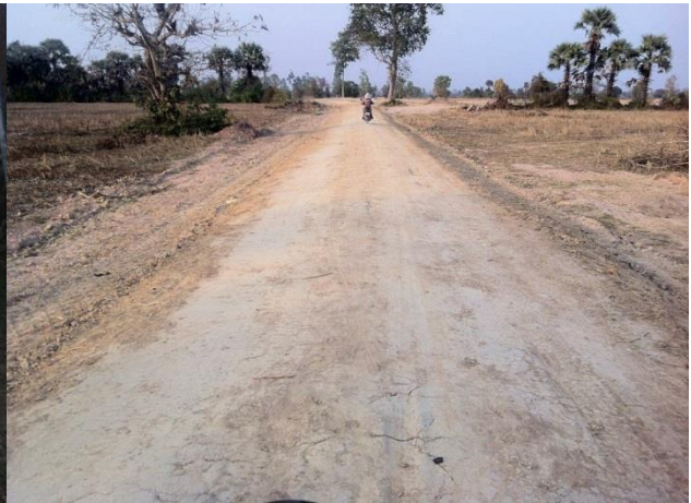
- Road construction (made from white soil) implemented 2015
